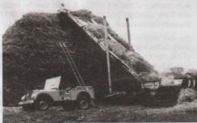
On the 15th of October 1947, the vehicle was sent to work. Here it is driving a Massey-Harris conveyor from its PTO
