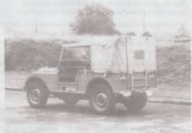
The completed Centre Steer Prototype photographed on the 15th of October 1947, complete with dummy capstan winch
